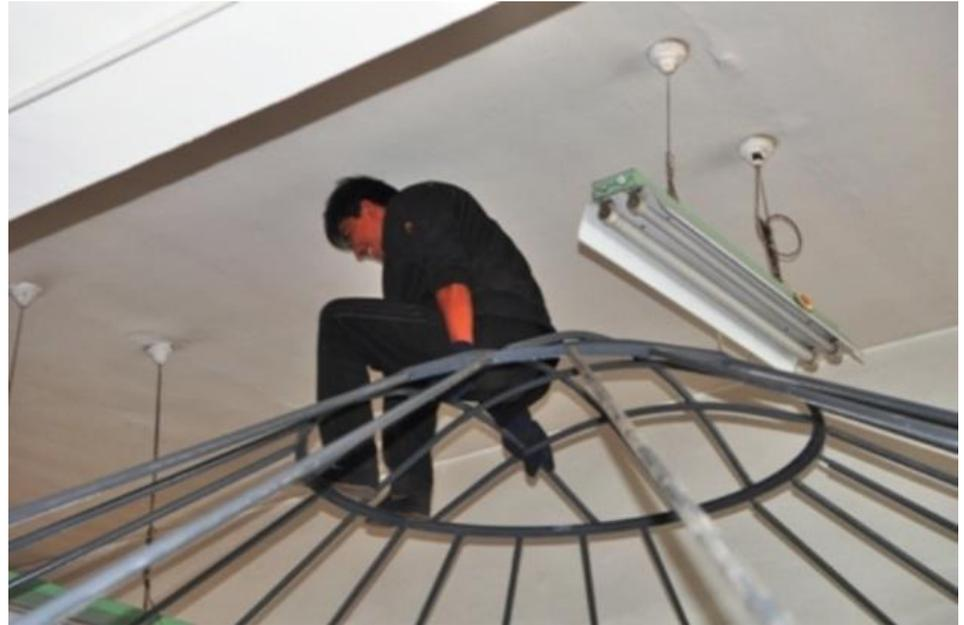
16) The crew using broomsticks help the **insulated top cover** move up the **rafters**. It will be a little heavy, it is insulated, and the larger the yurt, the heavier the cover. Be sure to have enough helpers on hand. >
