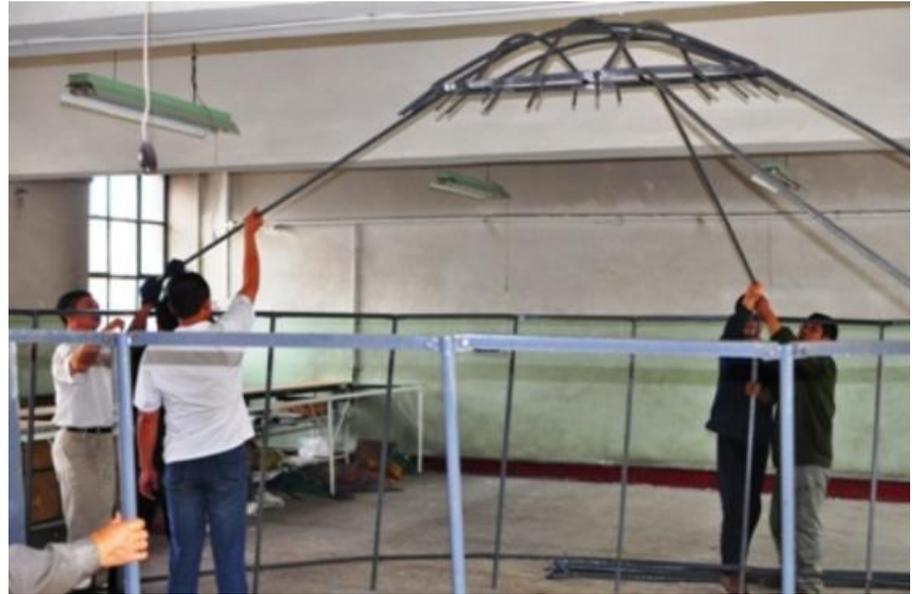
10) You can see here, a **rafter** slipped in the **wall support socket**. >
