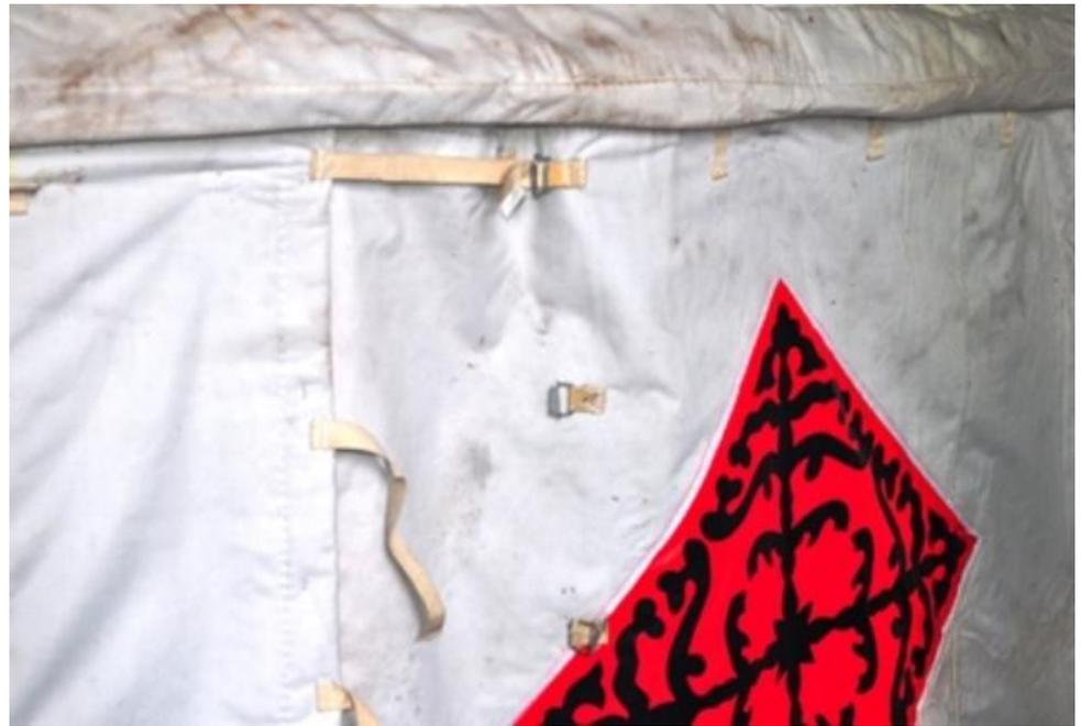
24) Next roll up the edge of the **insulated top cover**; this will expose the metal grommets made on the **insulated top cover** and wall loops sewn on the **insulated wall covers**. >
