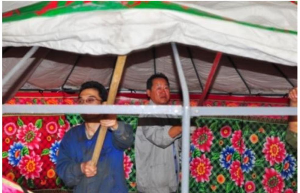
18) The hole in the **insulated top cover** needs to be centered over the outer ring of the **tono**. It isn't hard to do once it is on top of the **rafters**. >
