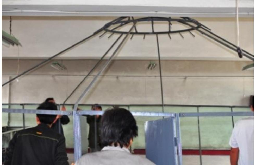
12) Pin the rest of the **rafters** and put them into the remaining **wall support sockets**. You may have to adjust the **wall supports** slightly to get the **rafters** to slide into place, but with the **rafters** fully in place, they should enforce a perfect circular space. >
