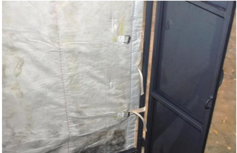
23) Use the outside straps and buckles in addition to inside ones to adjust the wall tension until it is firm, but not drum head tight. Now your insulated wall covers are in place and adjusted. Moisture and heat will make the walls naturally tighten or sag a little at times. >
