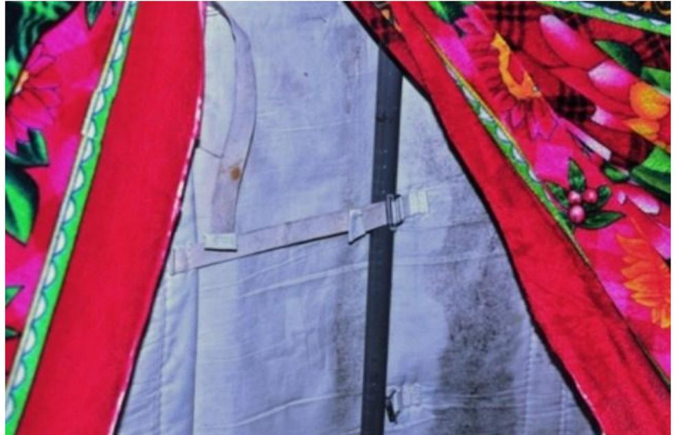
21) Additional straps and buckles are used to attach the **insulated wall cover** to the **batwing door** frame supports. >
